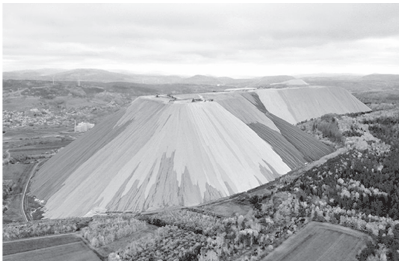
Figure 1. Potash tailings stack Kali mountain at Heringen, Germany [Photo: Vesna Pungercar].
